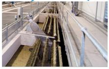
The Enflo-DAF<sup>TM</sup> rotary DAF scraper provides superior process and operational performance to the traditional "chain & flight" or "reciprocating bridge" type systems traditionally used for mechanical sludge removal.
