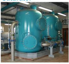
Enflo-DAF<sup>TM</sup> saturators are typically supplied as a pack-tower design, complete with internal media to provide transfer efficiencies greater than 90%, For industrial applications, unpacked saturators are also available. Saturators can be provided as mild (painted) or stainless steel vessels with internal surfaces being offered with scotch-coat finish or rubber lined.
